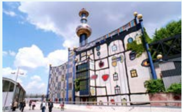
Spittelau Waste to Energy Facility, Austria
