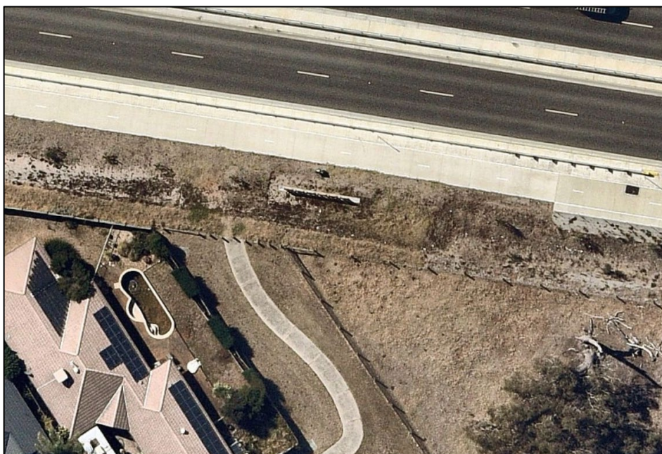
Figure 22 Unfinished footpath connecting Postregna Way and Hall Road (source: Nearmap)
