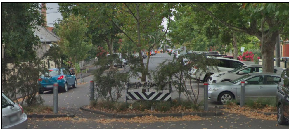
Figure 13 Example of a full road closure (from Google Maps Streetview)
