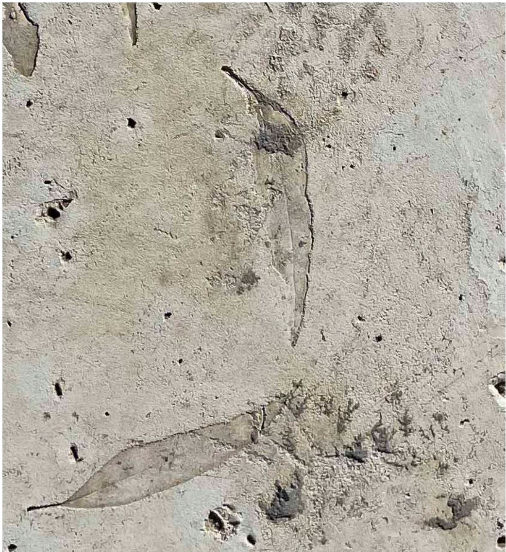
Concrete path finish with custom patterns
