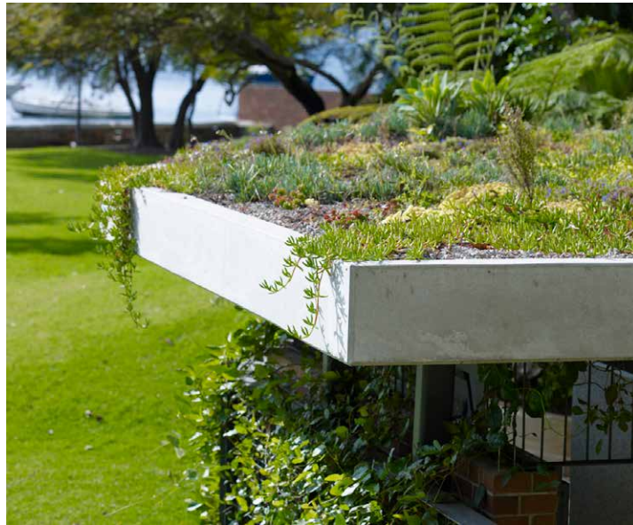
Figure 14: Green roof integrated with the amenity design in Beare Park, Sam Crawford Architects
