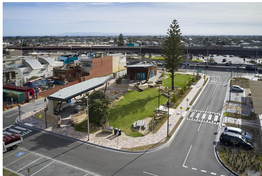
Carrum Level Crossing
