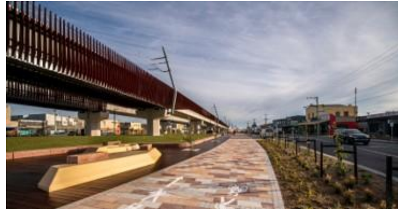
Carrum Level Crossing
