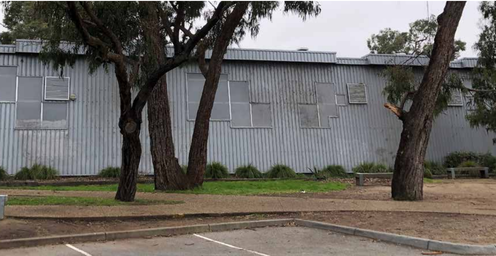
NARROW INTERFACE BETWEEN CAR PARK & PATHWAY WITH ERODING EXPOSED DIRT VISIBLE, SECTION OF PATHWAY TO BE REALIGNED WITH GARDEN BED PLANTING.. TWO EXISTING TREES REQUIRE REMOVAL BASED ON ARBORIST REVIEW
