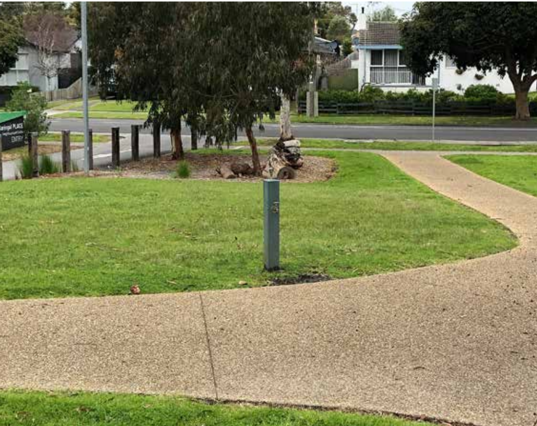
DRINKING FOUNTAIN WITH MUDDY BASE NOT ACCESSIBLE FOR WHEELCHAIRS TO BE REPLACED
