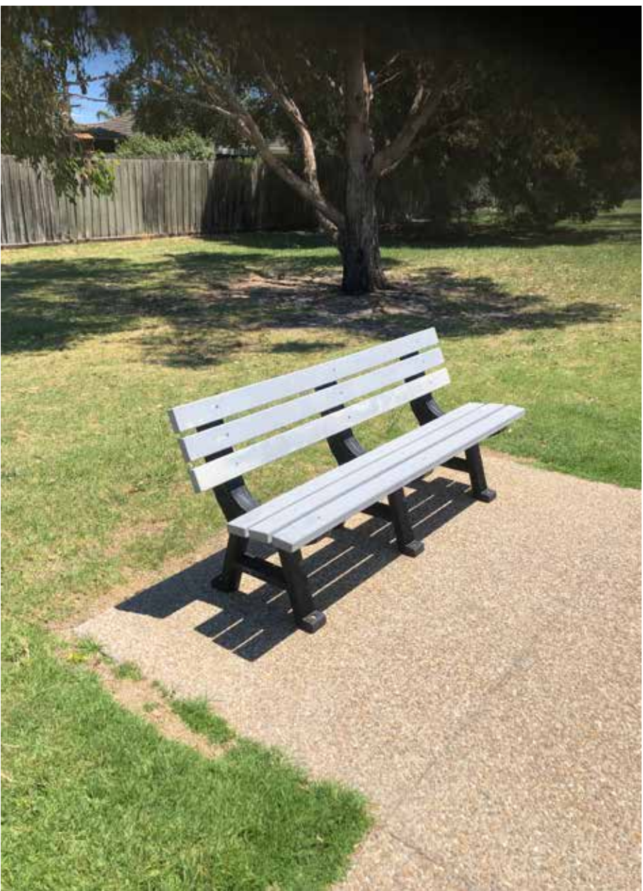
Existing park seats to be replaced
