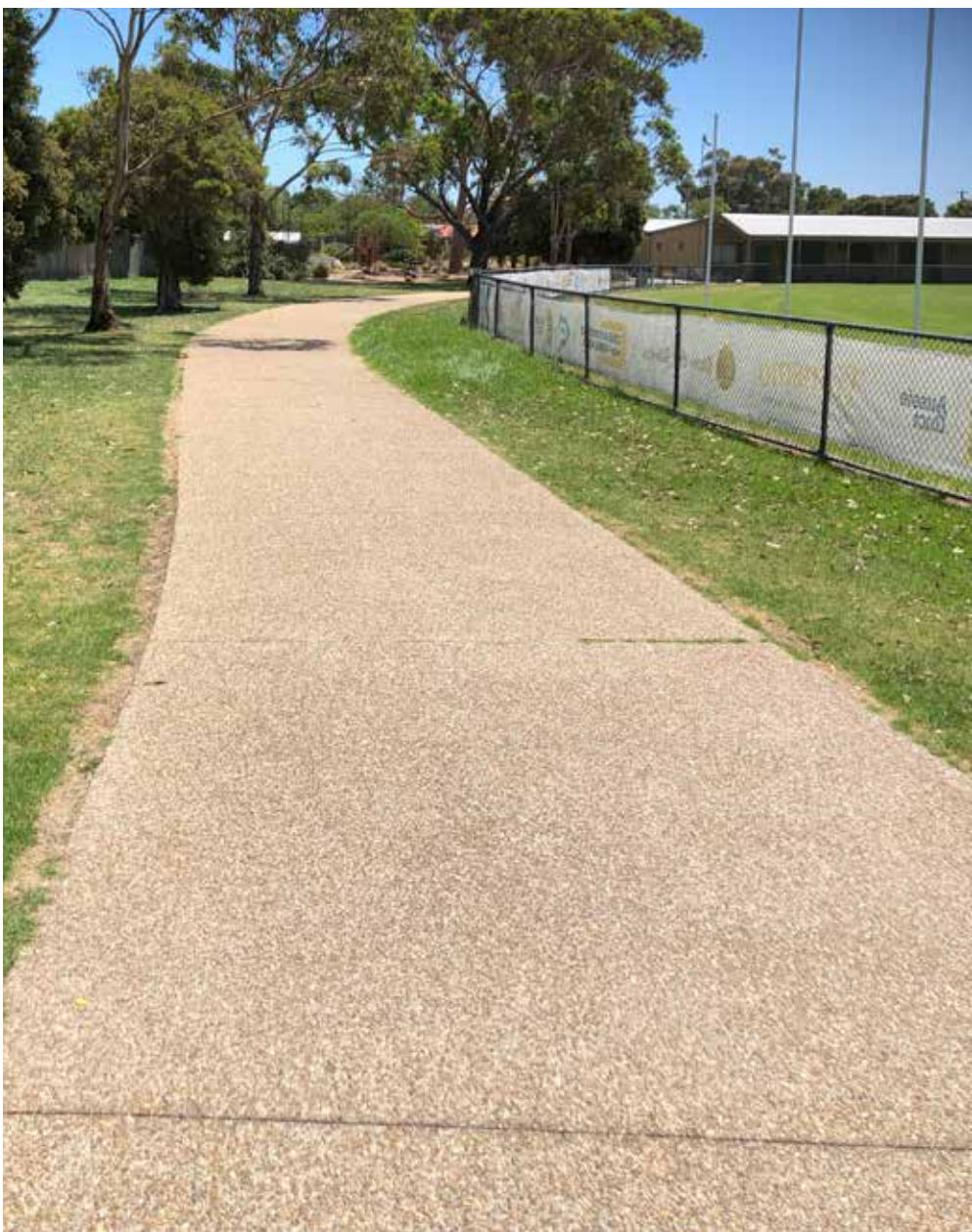
Sealed pathway to be retained.
