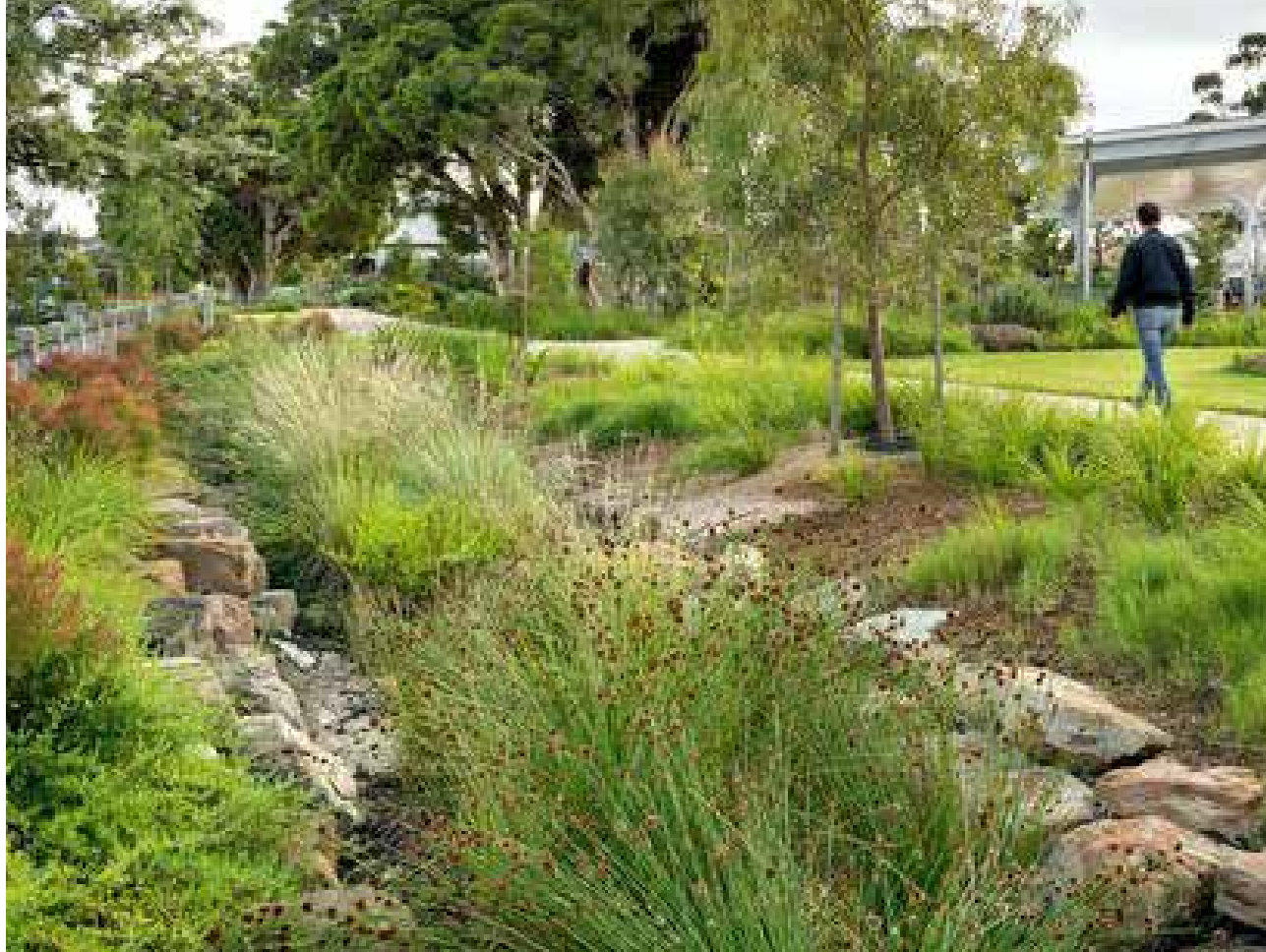
Native planted drainage swale
