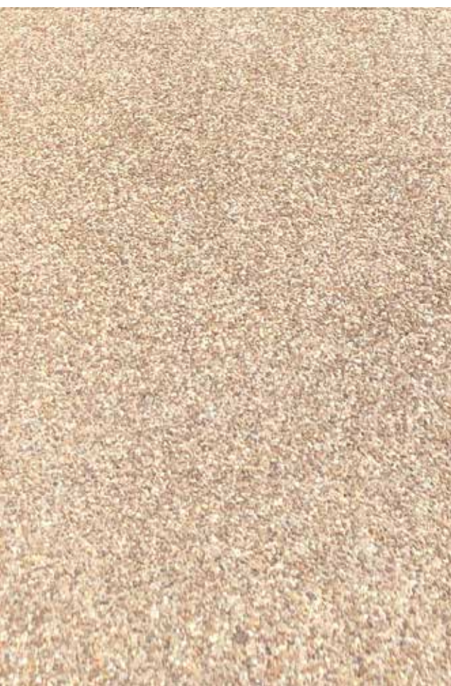
Coloured/exposed aggregate concrete for new pathway
